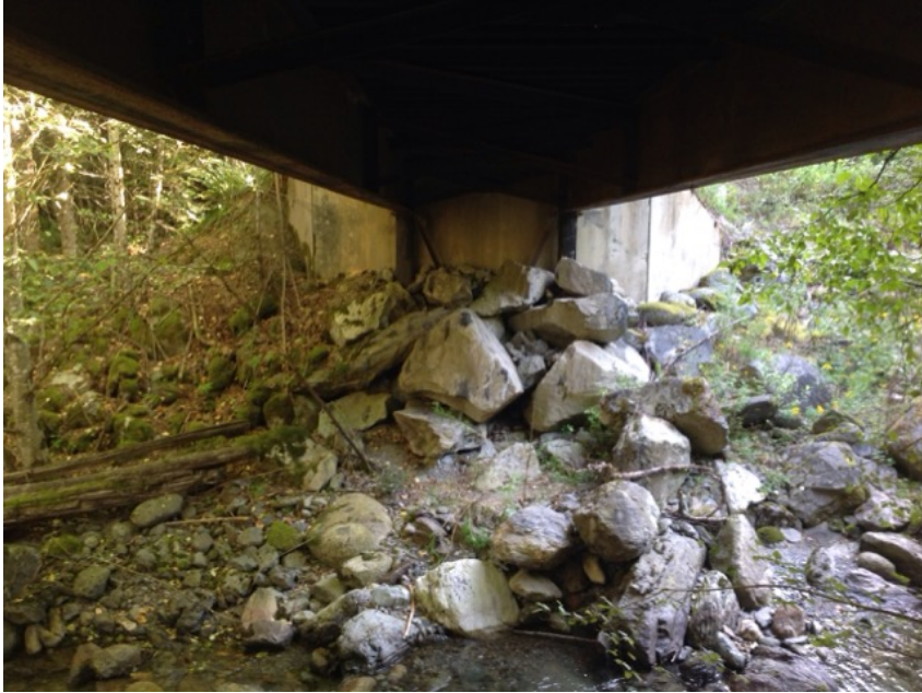
Right Bank Abutment when facing downstream
