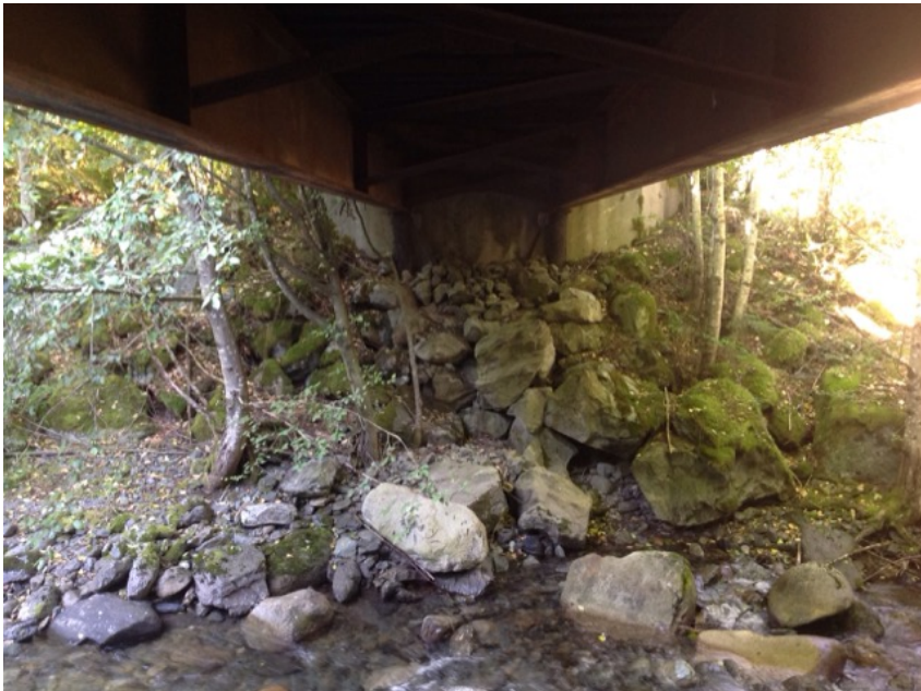
Left Bank Abutment when facing downstream
