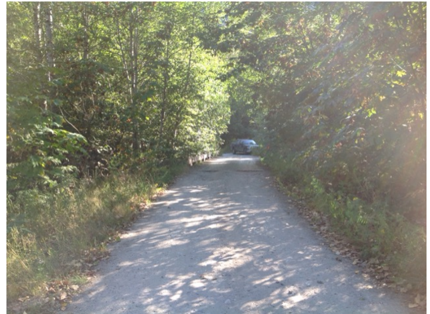
Approach from Left Bank when facing downstream
